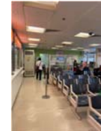
HEPA unit is placed at A&E area
