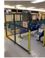
Temporary segregation on A&E area
